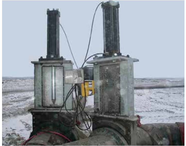
Cylinder position sensors operating in frigid arctic conditions to monitor pipeline valve actuators.
