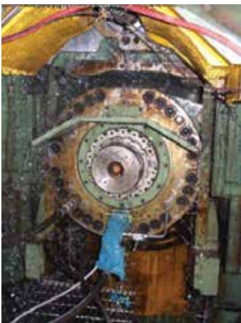
Production workaround to combat water ingress problems: blue plastic cover installed over a sensor in a steel rolling mill.
